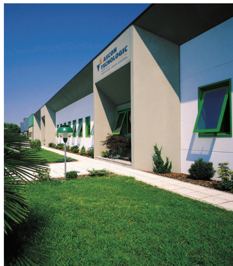
Headquarters, offices, R&D, Manufacturing unit, Vigevano (Italy).
